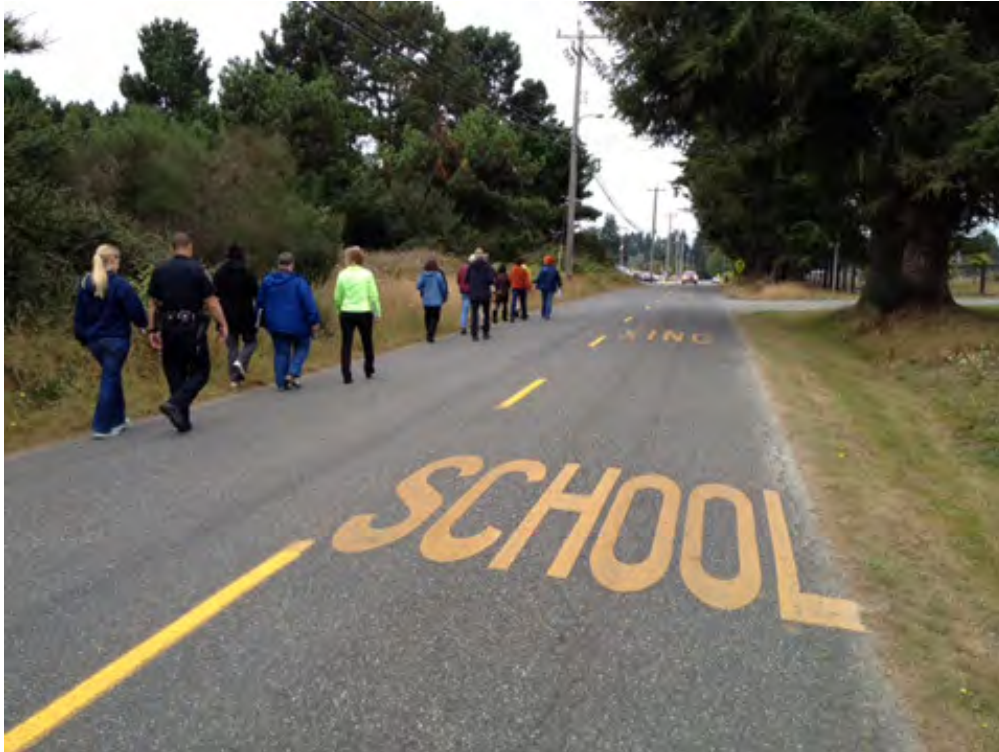
Pavement markings indicate it is a school zone, but the lack of sidewalks on Dow's Prairie Road is hazardous for pedestrians.
