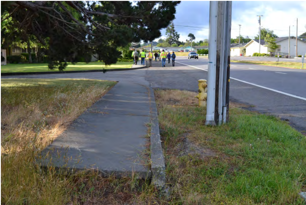
Sidewalks on Ross Hill Road are missing or not connected
