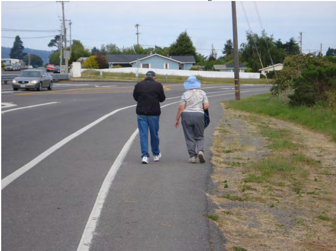
Pedestrians don't feel safe when cars drive quickly around this curve on Ross Hill Rd.
