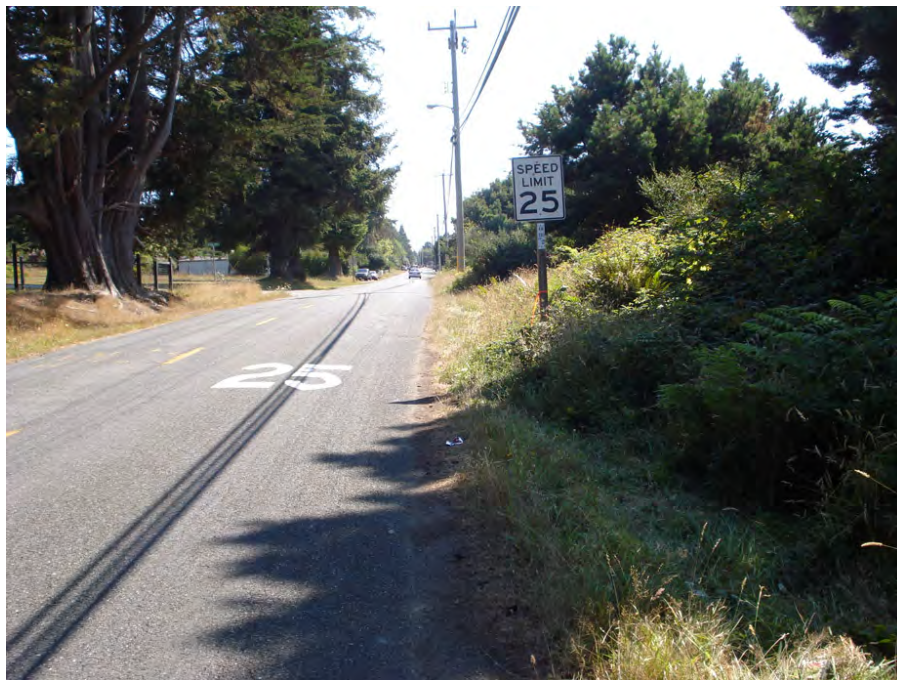
The overgrowth of brush contributes to poor sight visibility and forces pedestrians to walk further out into the street.
