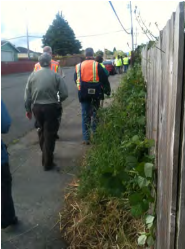
Vegetation is encroaching upon the sidewalk on Wood Street.
