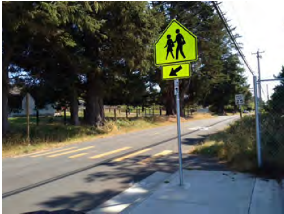
The sidewalk in front of the school ends at the south end of the parking lot. Without sidewalks on the east side of the street, this crosswalk leads to a ditch.
