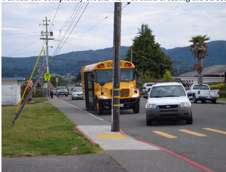
Extending the red curb (No Parking Zone) could increase visibility at this crosswalk.
