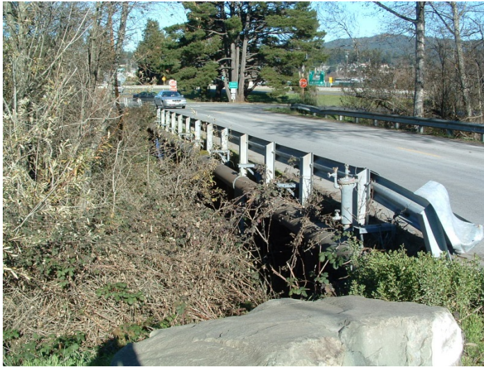
Figure 31: Strongs Creek Bridge on Riverwalk Drive - Looking East
