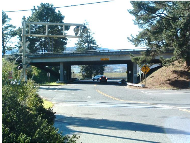
Figure 32: Kenmar Road Undercrossing Looking West
