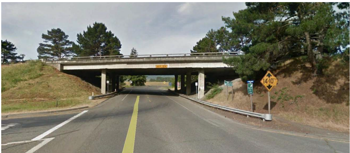
Figure 5: View of Kenmar Road Undercrossing
