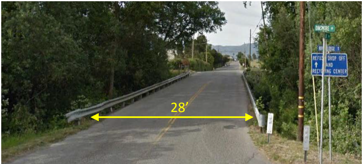
Figure 52: Strongs Creek Bridge on Riverwalk Drive, Looking South
