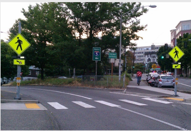
RRFB lights/sign. User-activated “rectangular rapid flashing beacon” (RRFB) at major crossings
