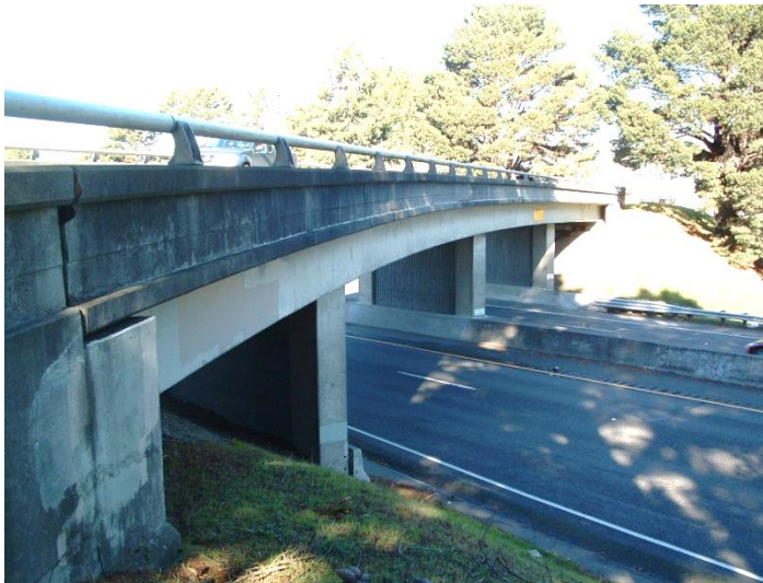
Figure 29: 12th Street Overcrossing - Looking East
