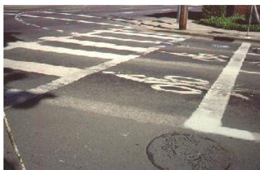
Bike box in Eugene, OR. (Photo: Evaluation of an Innovative Application of the Bike Box, FHWA, 2000.)
